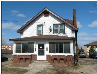
Front porch for lower unit
