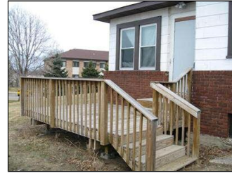
Deck for upper entrance
